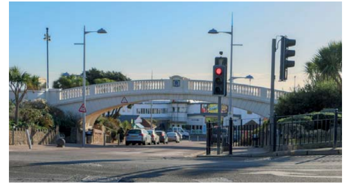
Figure 21 Pier Gap Bridge (looking South)
