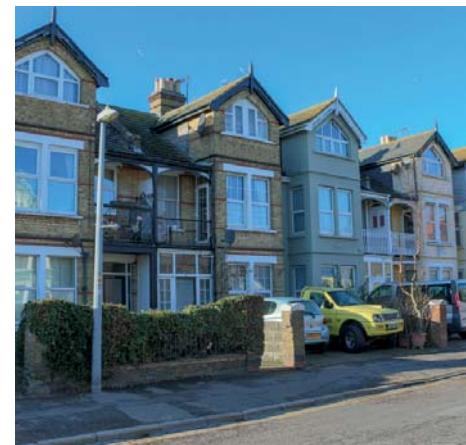
Figure 41 Agate Road (looking West)
