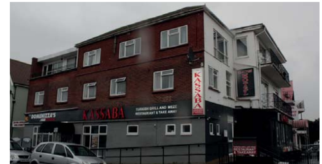
Figure 18 Example of inappropriate signage and paint colour on West Marine Parade
