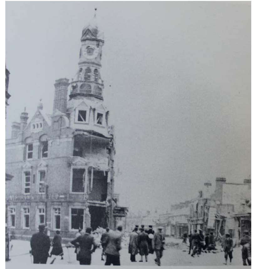
Figure 12 Air Raid Damage 1941 (Britain in Old Photographs 1995)
